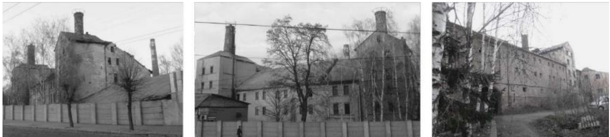
Fig.1. The current condition of the brewery
